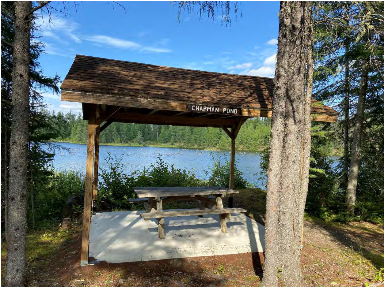
Figure 15. View of recreational area at Chapman Pond (installed by Eagle Scouts in 2016 according to the cement foundation).
