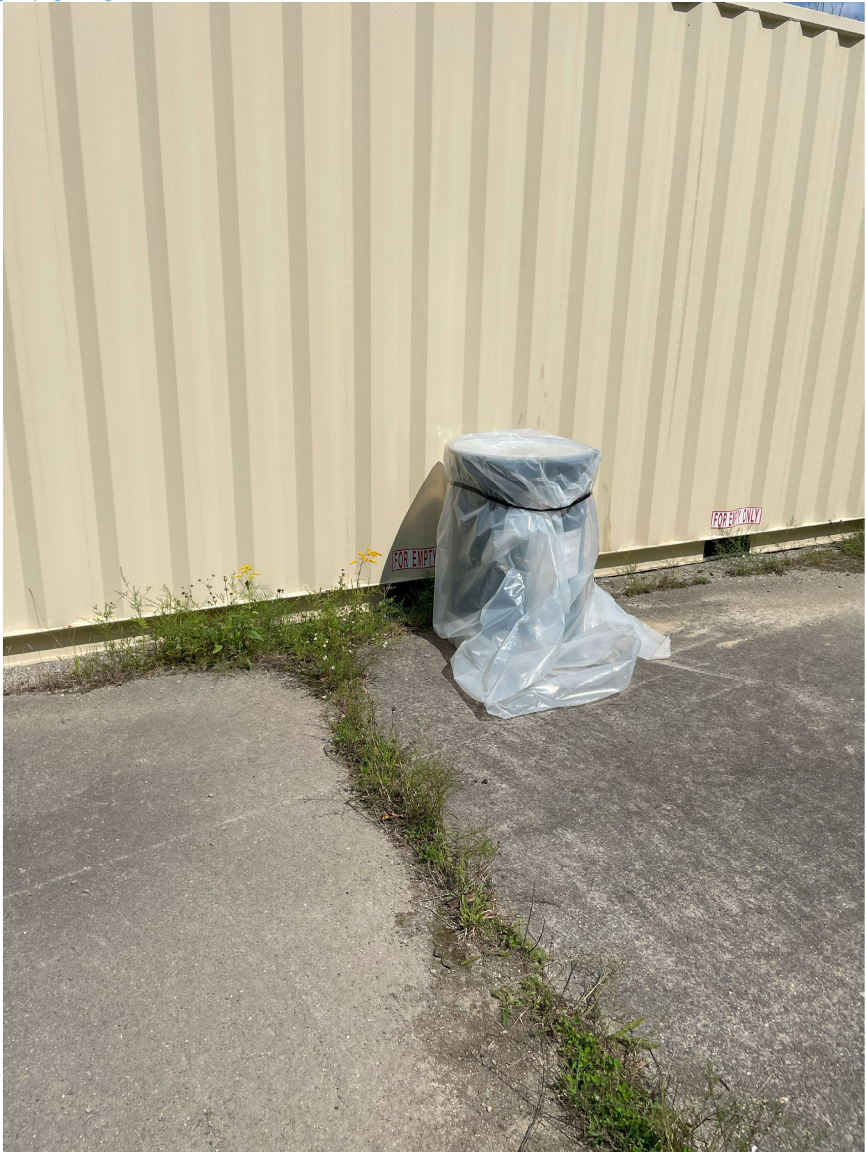
PHOTO 001: IDW drum consisting of soil cuttings from the direct push technology (DPT) soil investigation. Drum staged next to connex trailer and secured with plastic wrap.
