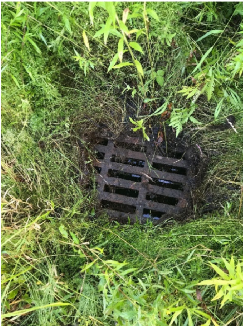
Catch basin was filled to grade with stormwater.
