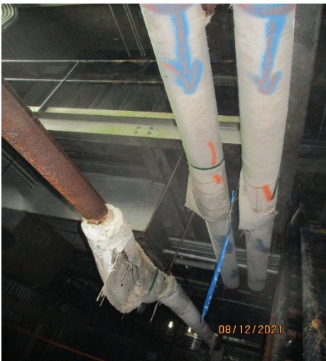
Photo 1&2-25: Non-ACM by Analysis
