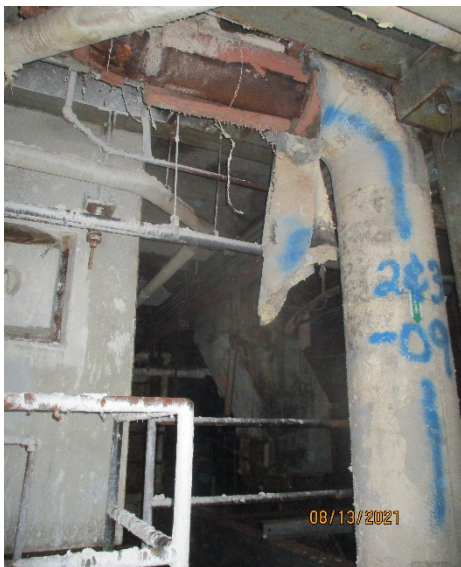
Photo 3&4-09: Positive ACM by Analysis
