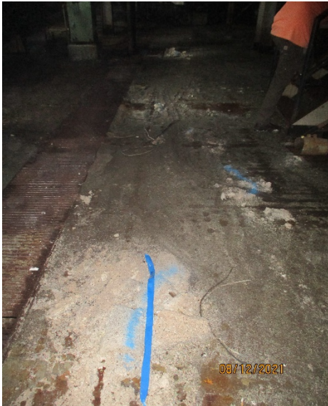
Photo 1&2-27: Non-ACM by Analysis
