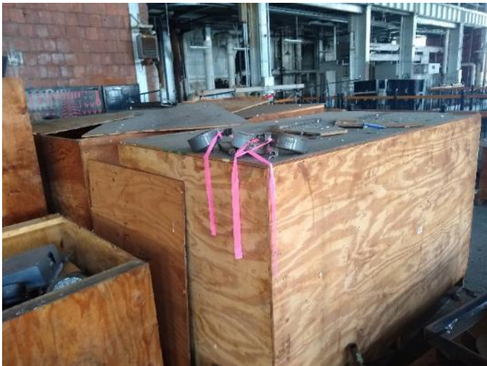
Location M16: View of three Mercoïd® switches and one thermometer all still containing mercury. Centrally located second level.
