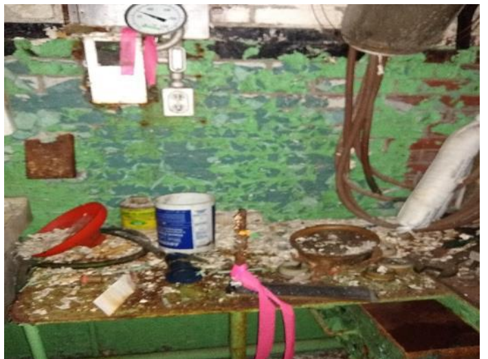
Location M04: View of two (out of three) mercury containing thermometers located within the maintenance shop on the ground level.
