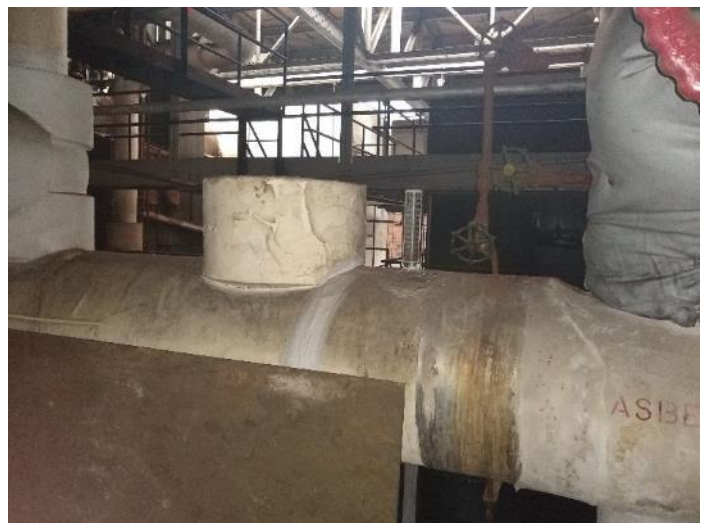
Location M18: Mercury thermometer attached to #3 boiler.
