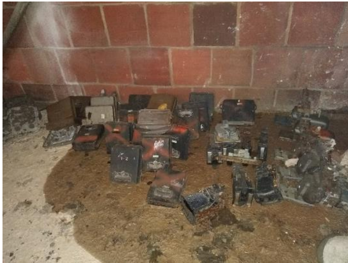
Location M20: Various Bailey Meters and other equipment that formerly or currently contain mercury.
