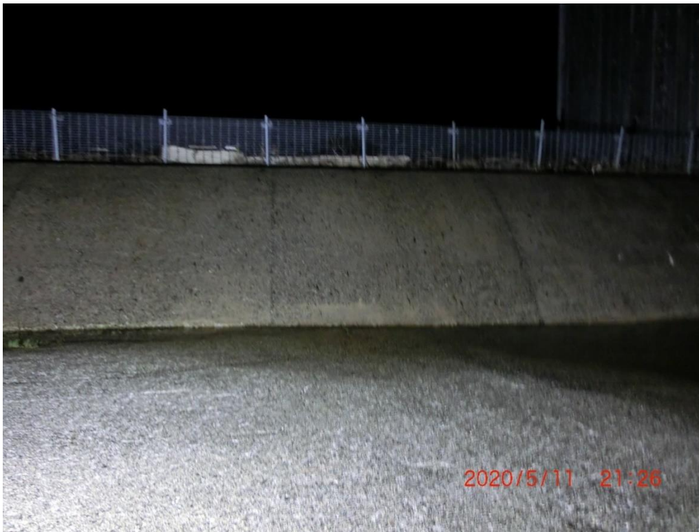
Photo 7-8 – Looking for eels at night – spillway
