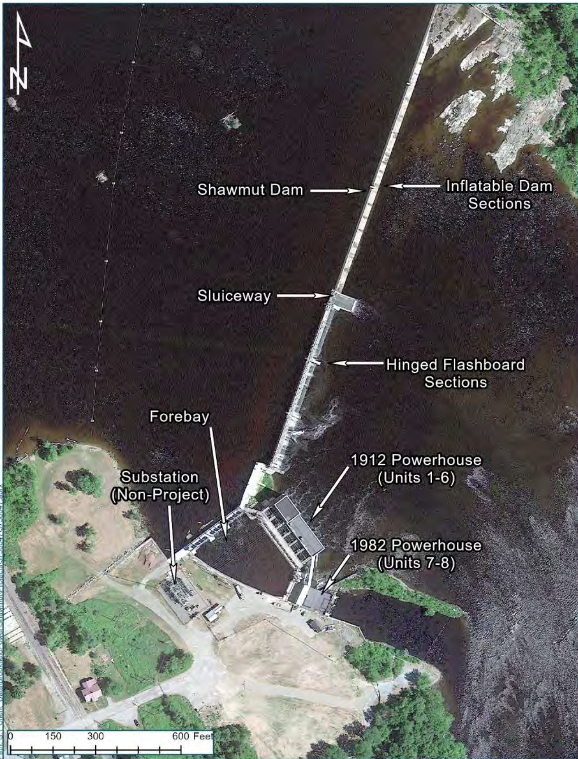
Figure 3-1 Overview of Shawmut Project Facilities
