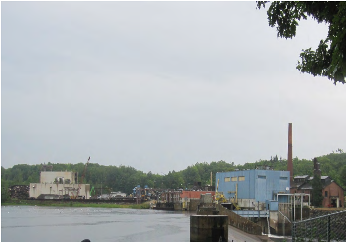
Figure 4.10.1.1-3. View of Powerhouses and Grimm Industries
