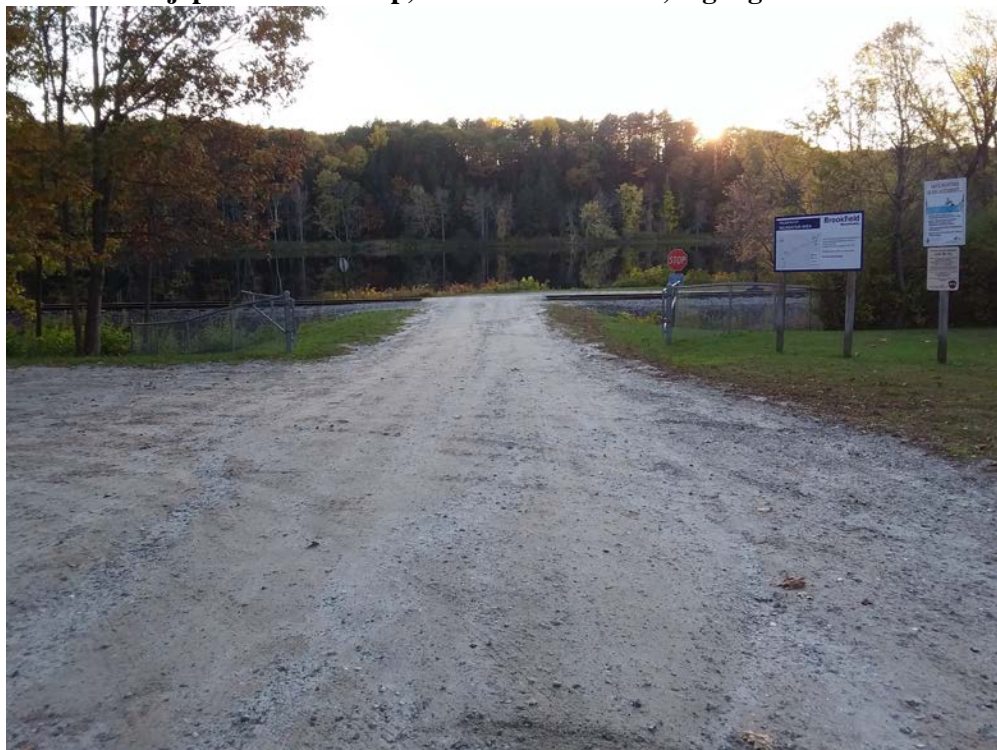
(Photo taken by M. Rheume, Gomez and Sullivan Engineers, 10/15/2019)
