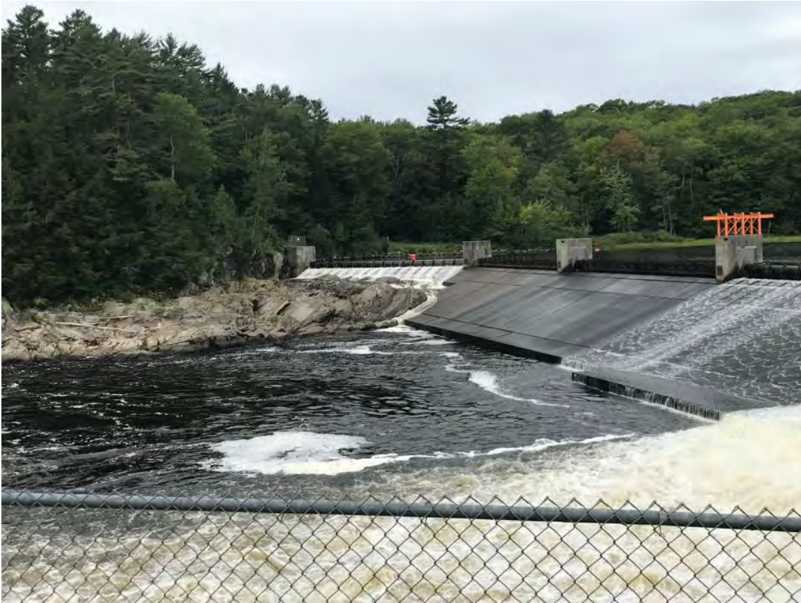
Figure 4.6.1.3.2-1: Initiation of Bascule Gate Operation
