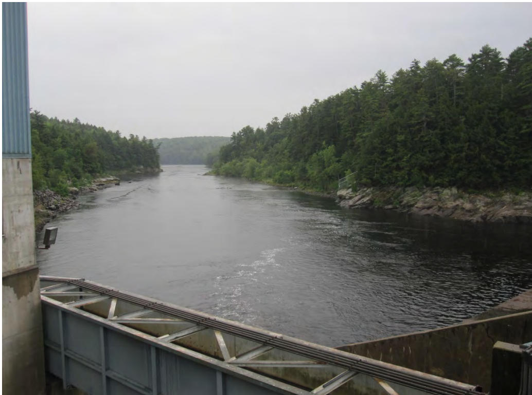
Figure 4.10.1.1-1. View Looking Downstream from Pejepscot Dam
