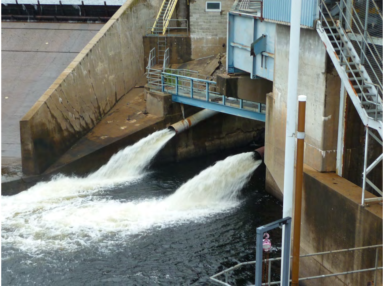
Figure 2.1.3.2-2: Downstream Fish Passage Facility Transport Pipes
