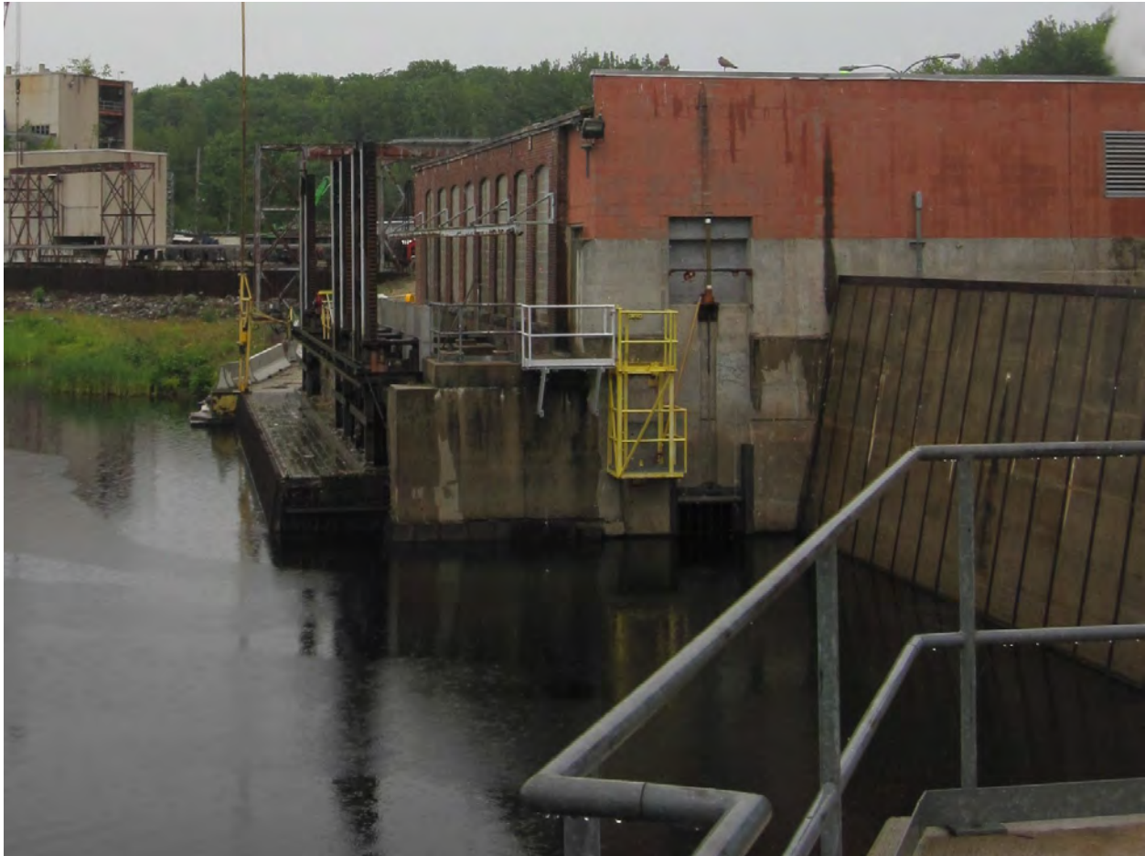
Figure 2.1.2-1: Original Powerhouse and Intake
