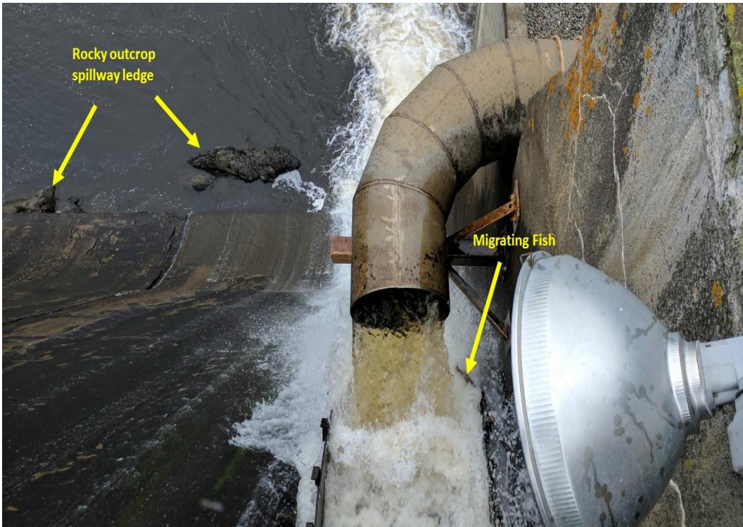
Figure 20. Spillway flume and downstream migrant pipe at Ellsworth Dam. (Source: FERC).
