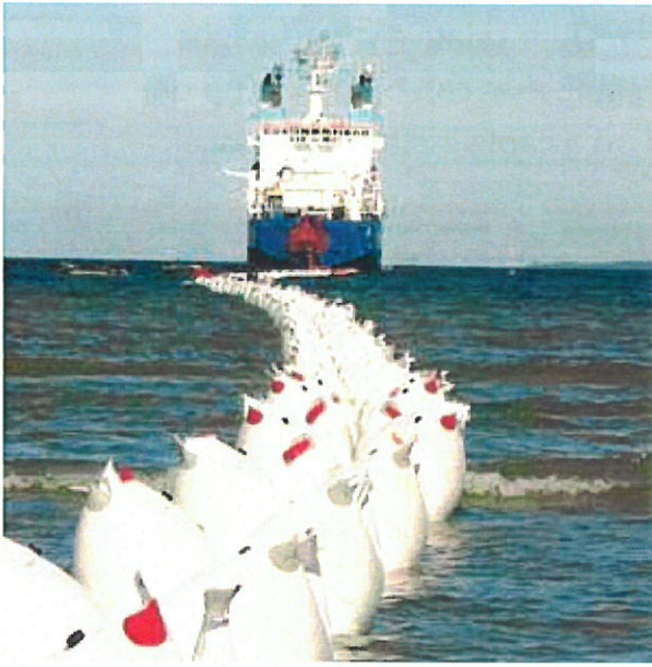
Photo 5 -- Laying the Estlink HVDC Light cable 2x75 km. HVDC Light cables can connect two countries or offshore wind farms by undersea. (photo courtesy of ABB)
