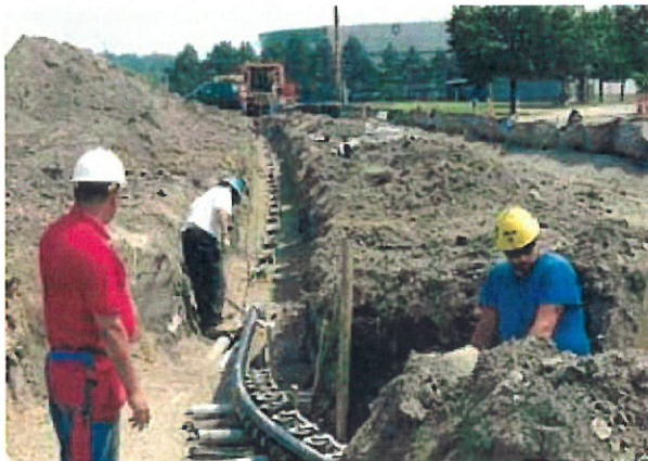
Photo 4 -- Laying HVDC Light cable in New Haven, Connecticut. (photo courtesy of ABB)
