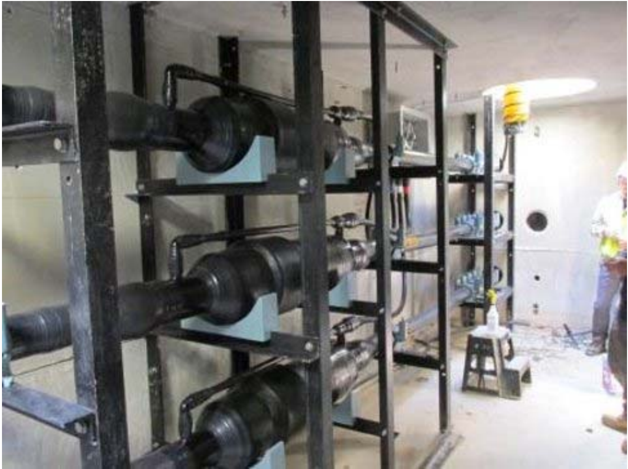
Figure 15 - Cable Joints in Vault
