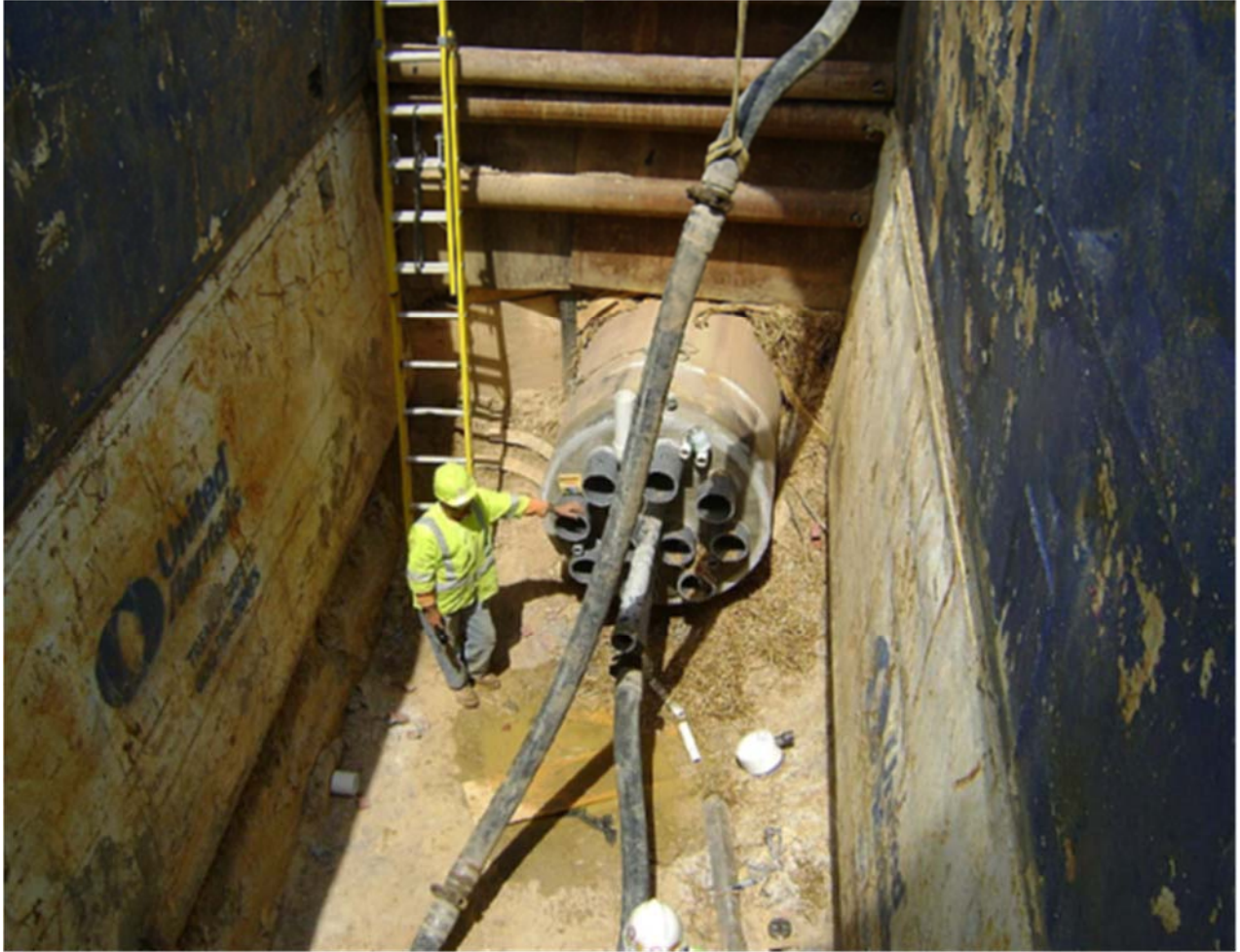
Figure 9- Pipe-Jacking Shaft
