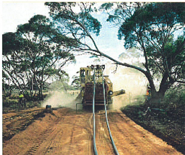
5 Construction of Murraylink HVDC Light® (Australia).
