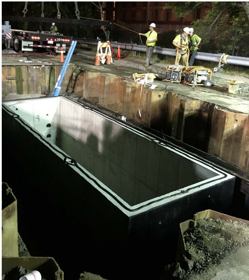
Figure 4- 115kV Splicing Vault
