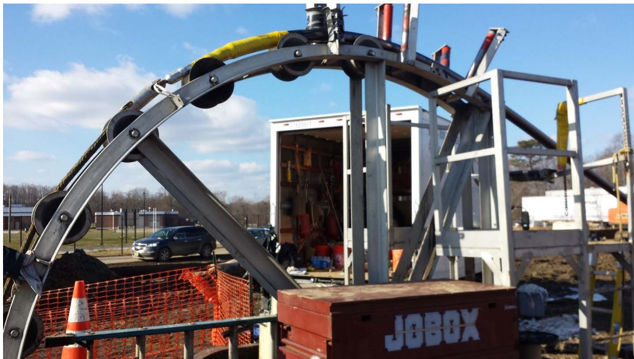
Figure 12- Cable Pulling over Bullwheel
