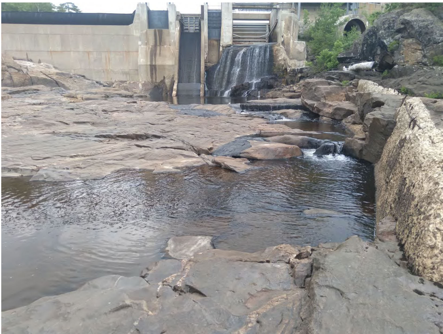
Photo 2, East side 2: This photo shows the gates up close, with about 100 feet of river bottom. It demonstrates all the more starkly the scouring effect of releases from the dam gates on the substrate of the river in this section.
