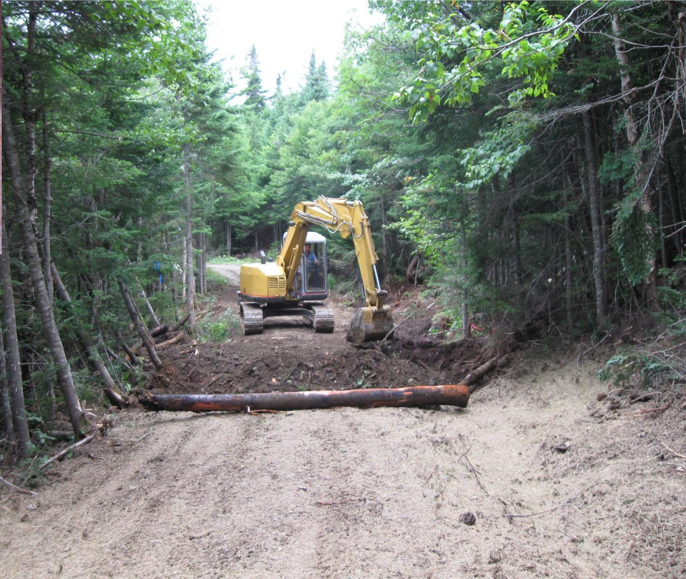
Proper ditching and drainage is necessary for trails to be sustainable.
