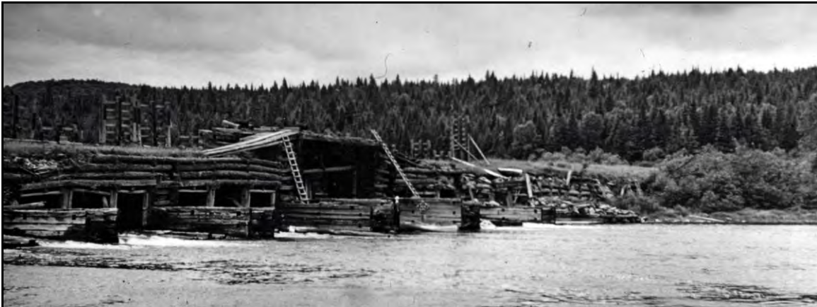
(Above) 1957 Al Mitchell Photo of the No-Longer-Standing Long Lake Dam
