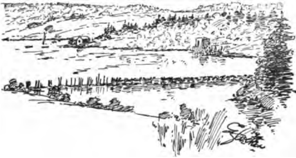
OLD DAM, McCAFFREY'S CREEK
