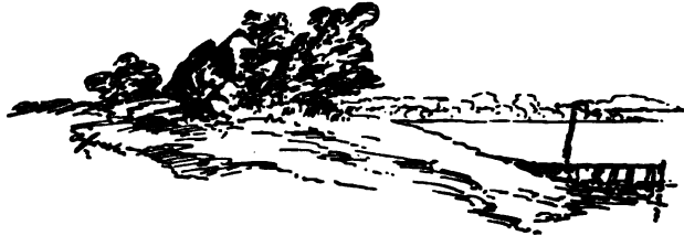
FORT FREDERICK BEFORE THE EXCAVATION
