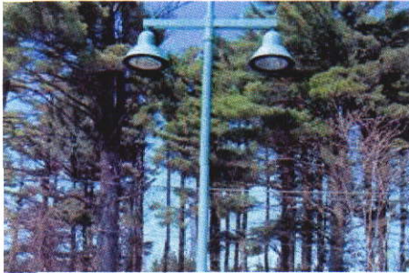
An example of well- shielded lighting.
