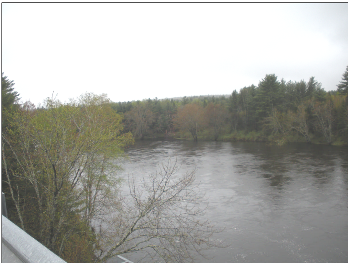
Springtime view of the Piscataquis River from Trestle Bridge. May 2011
