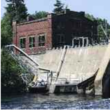
Fort Halifax dam, Kennebec River
