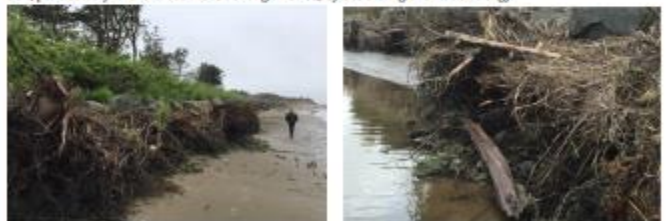
Figure 1. Root wads inserted into unstable banks can help protect bare soil from erosion, from a project in coastal Oregon. In areas not suitable for living shorelines, root wads can be an effective alternative providing stabilization and habitat.
