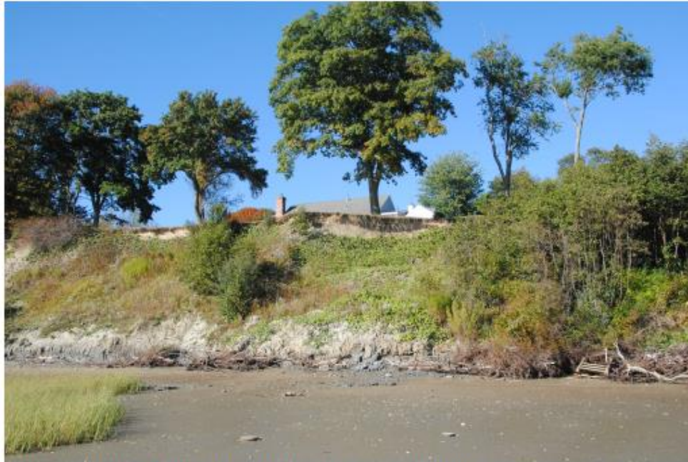
Bunganuc Bluff, Brunswick, ME. Newly visited site with a direct concern for private property. Site of a recent major rotational landslide (not included in photo). Highly unstable and expected to fail in near-time.
