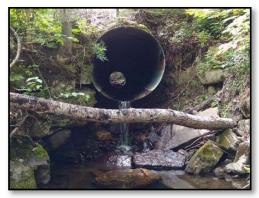
Narrow culverts become perched, preventing passage of fish and wildlife and backing up during high water events.
