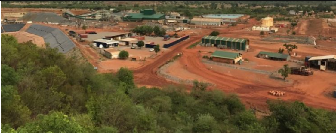
An overview of the Perkoa mine site, Burkina Faso, pictured in a Trevali Mining Corporation technical report. Photo: trevali.com
