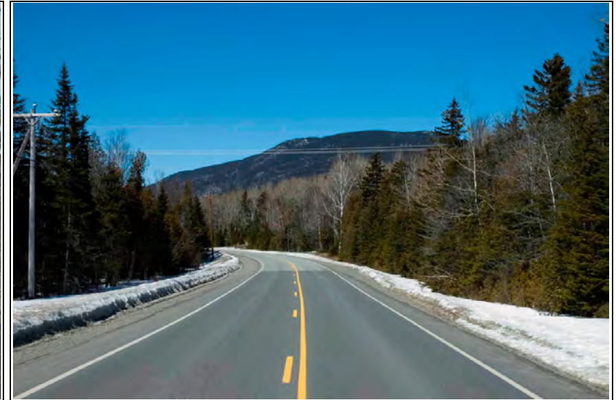
Photo 20b. Route 16/27 115kv Crossing Looking North Only the wires are visible at the crossing of the existing Boralex line; poles would be similarly set back from the road with the proposed line.
