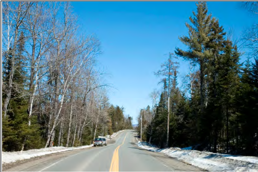
Photo 20c. Route 16 Transmission Crossing Looking North.
