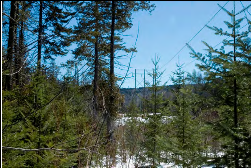
Photo 20a. Existing Boralex 115kv Transmission Line At AT Crossing Most plantings are very dense and the line is difficult to see. The proposed line would be similarly screened
