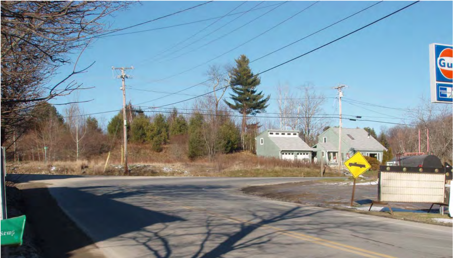
Southern Segment: Intersection of Route 1A and Franklin Center
