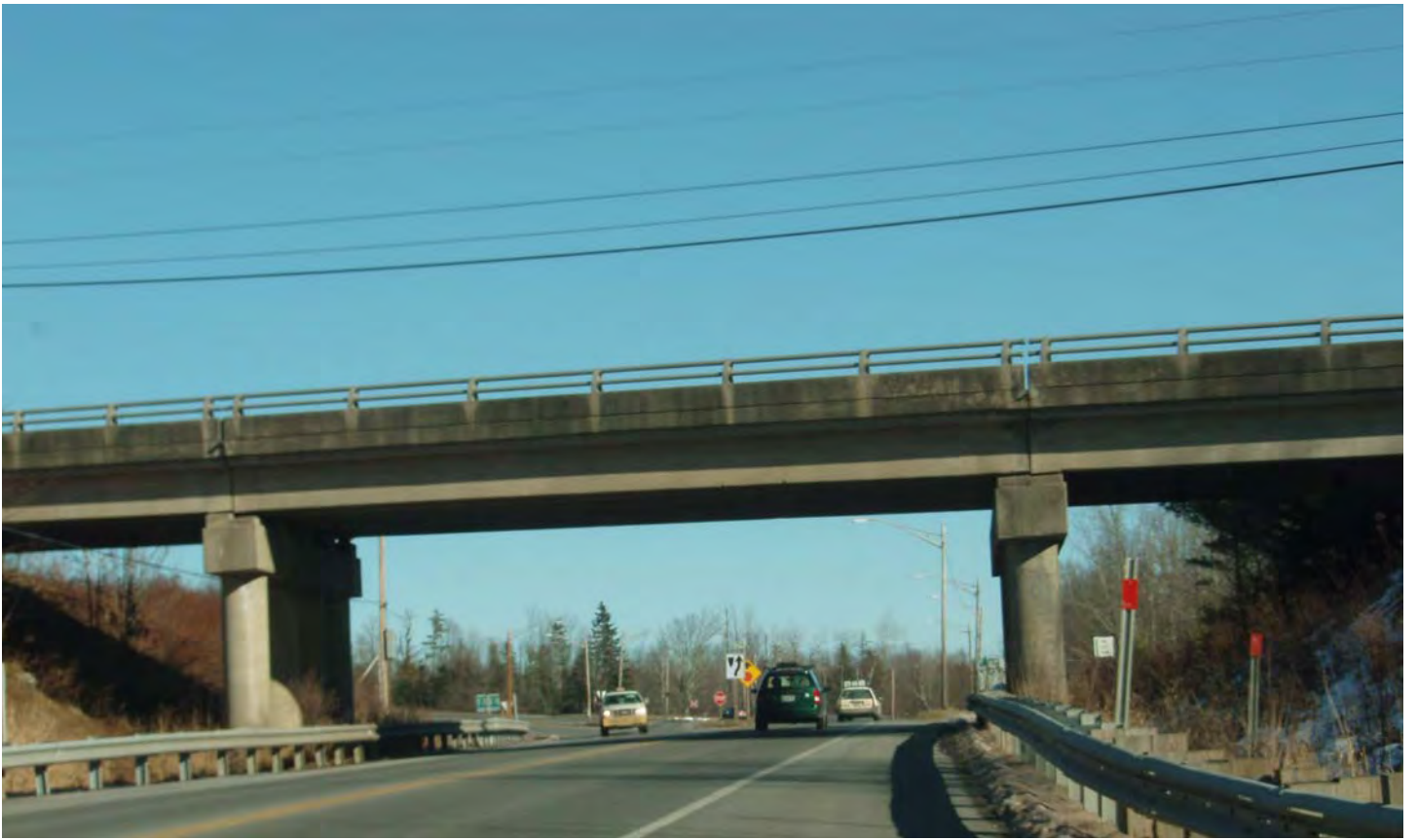
Southern Segment: Bridge over Route 1 near Route 1A Diverge
