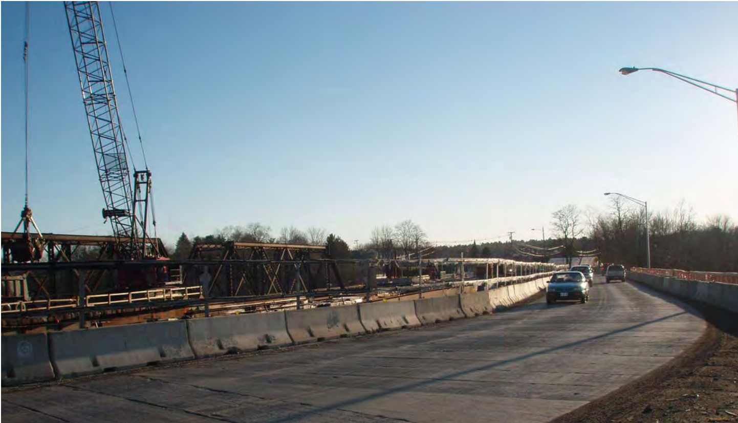
Central Segment: Route 2 Bridge Reconstruction over the Penobscot River
