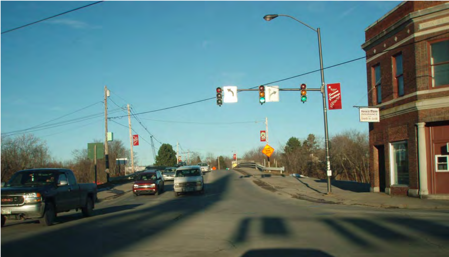
Central Segment: Route 2 Bridge over West Branch of Penobscot River
