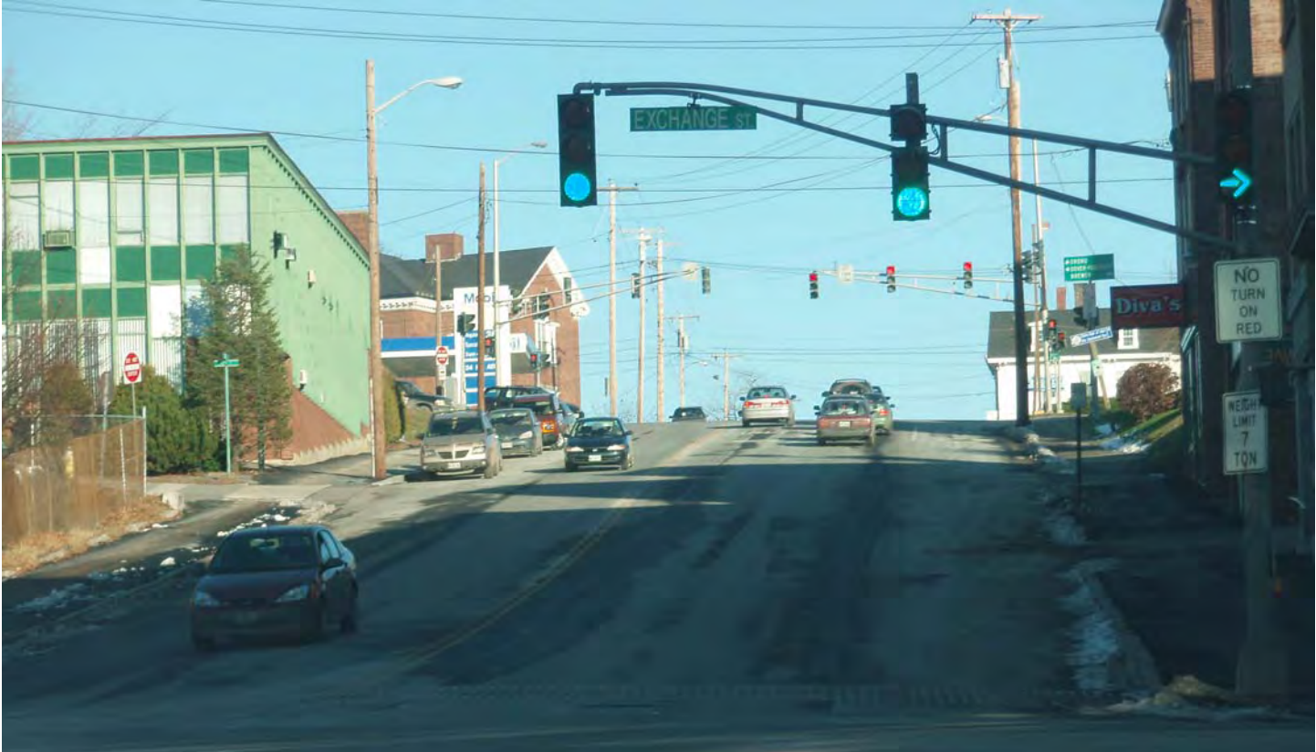
Central Segment: Steep Grade on Route 2 (State Street)
