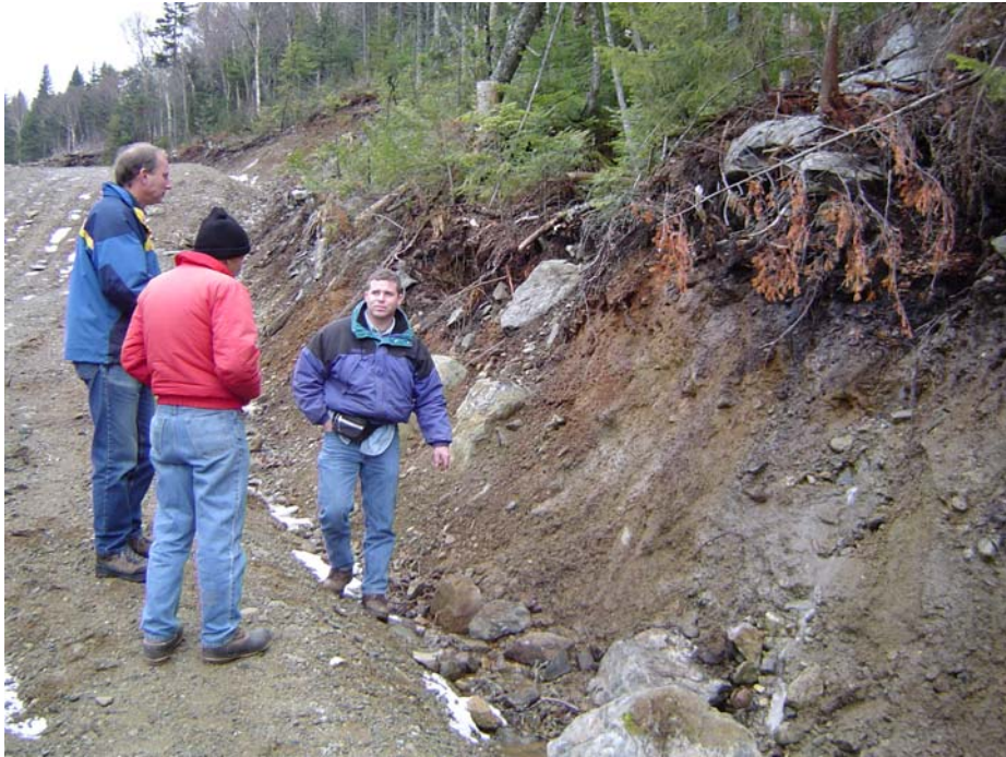
Photo 8: Boulders and cobbles encountered on surface shall be utilized to downslope fill extensions. Photograph by Albert Frick, 11/12/2003.
