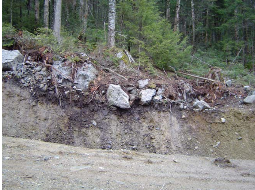
Photo 2: Existing high elevation road cut at Seven Ponds TWP at 2,600' +/-. Photo illustrates typical strong surface horizon over glacial basal till substratum. Location not in project area, however, used as available example of deep road cut in high elevation mountainous area, exhibiting typical very stony soil surface over firm basal till. Photographer A.F. 11/12/2003.
