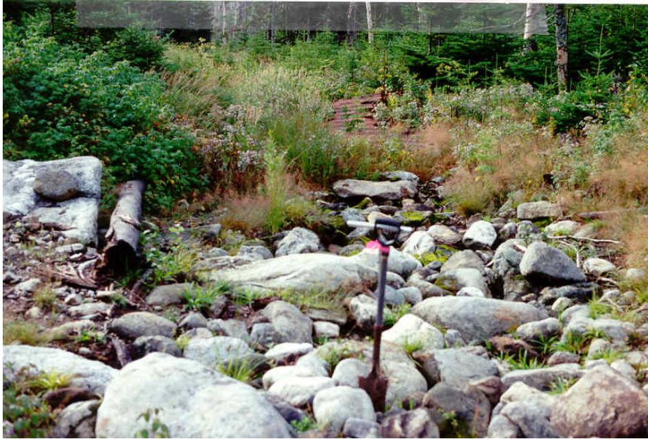
Photo 1: Extremely stony surface phase encountered in segments of proposed road on Redington Ridge. Photographed by A.F. 8/22/2003.
