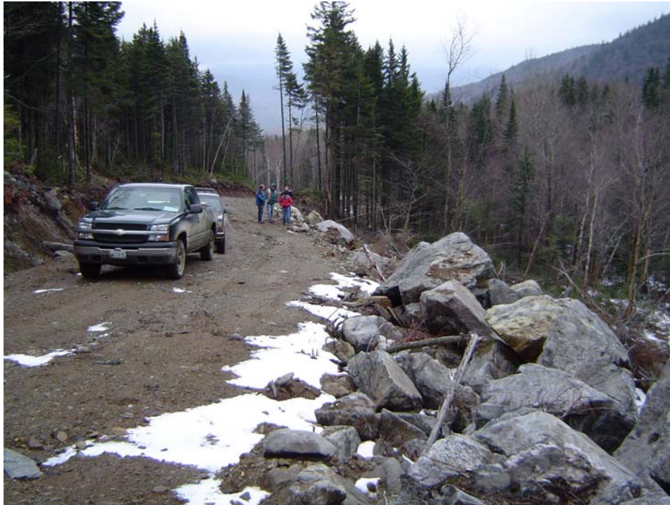
Photo 10: Armored downslope road fill extension, 11/12/2003.
