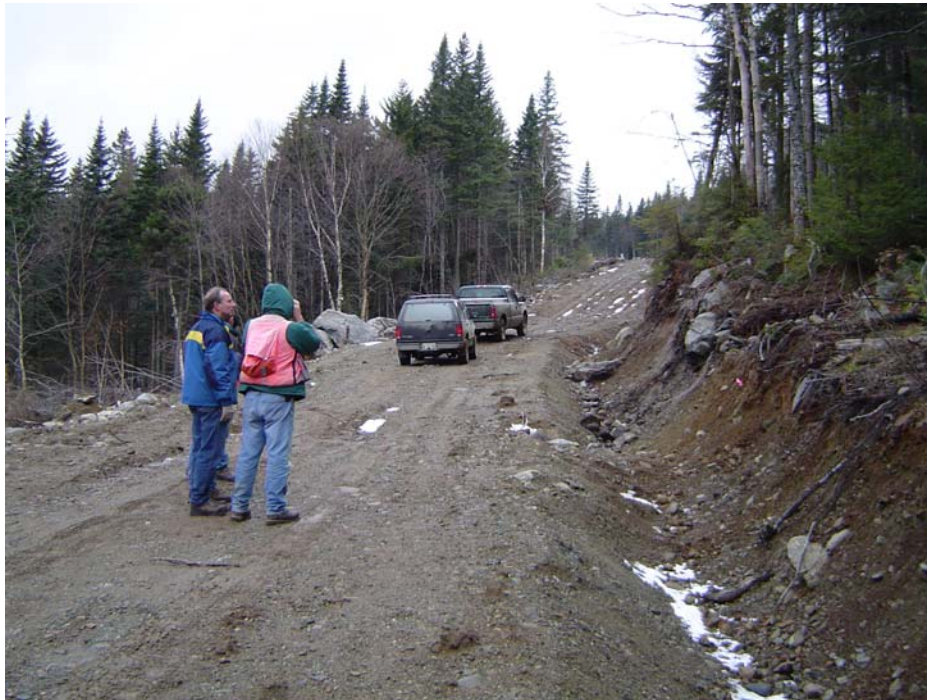
Photo 11: View of existing 14% road grade, which is typical upper tolerable design limit. Photograph by Albert Frick, 11/12/2003.
