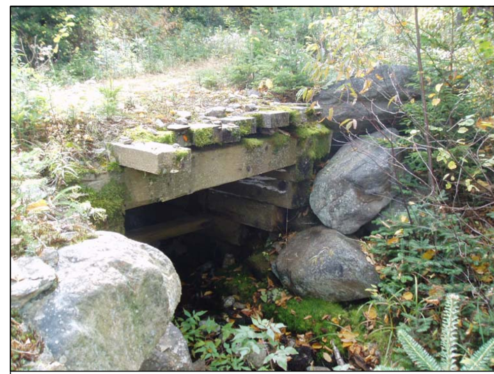
PHOTO 1 - TAKEN LOOKING SOUTHERLY AT WOODEN BOX CULVERT
