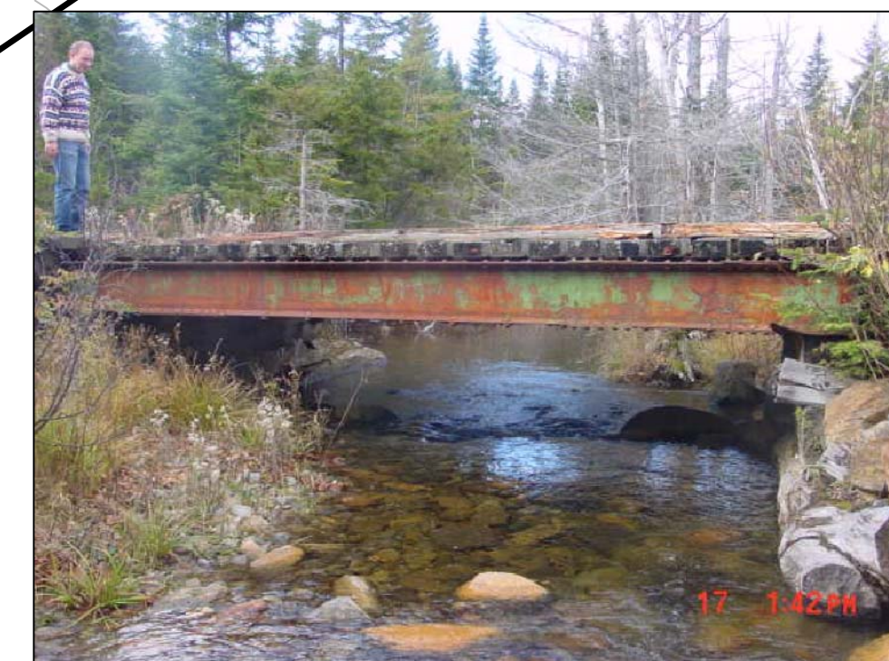
PHOTO 2 - TAKEN LOOKING NORTHWESTERLY AT EXISTING STREAM CROSSING
