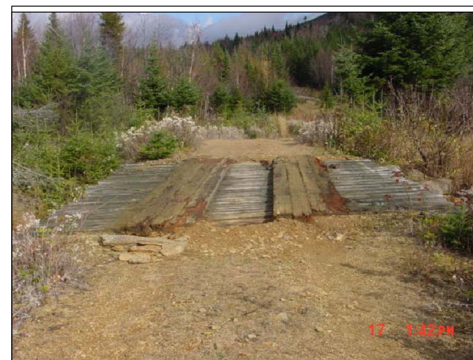
PHOTO 1 - TAKEN LOOKING NORTHEASTERLY AT EXISTING STREAM CROSSING
