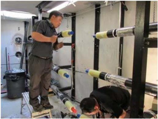
Figure 13 - Preparing Cable for Jointing
