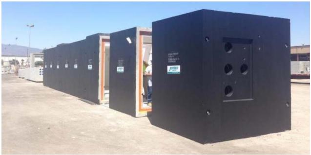
Figure 3 - 500kV Splicing Vault
