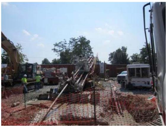
Figure 6 - Horizontal Directional Drill Rig
