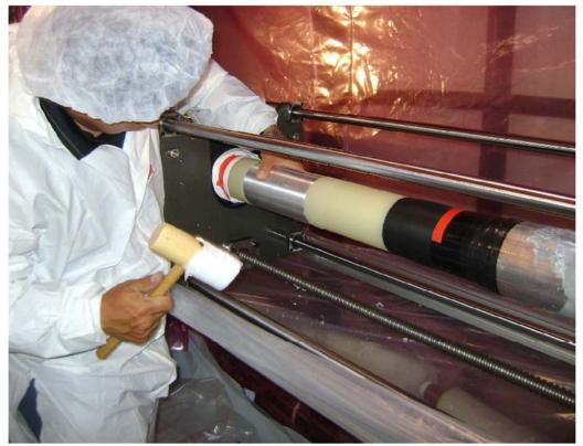
Figure 14 - Assembling Joint
