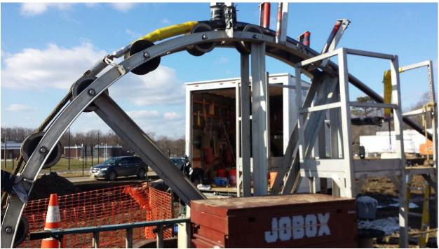
Figure 12- Cable Pulling over Bullwheel
