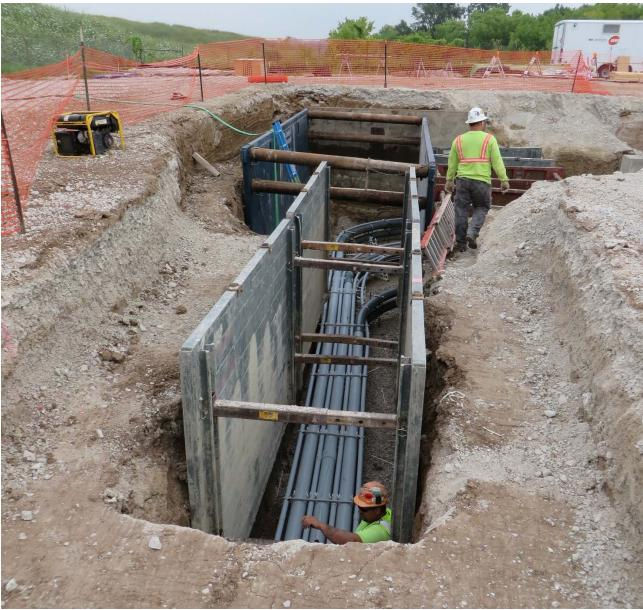
Figure 2- Duct Bank Excavation
