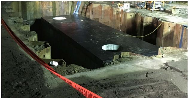
Figure 5- 115kV Splicing Vault
