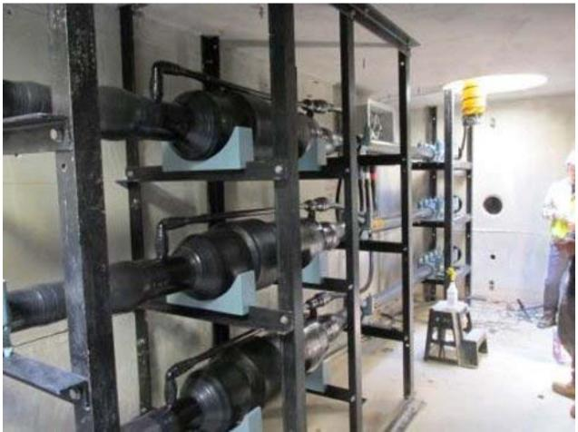
Figure 15 - Cable Joints in Vault
