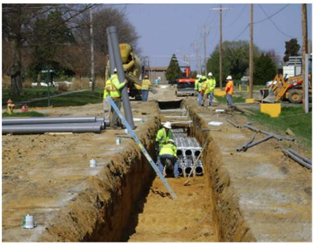
Figure 1 - Duct Bank Excavation
