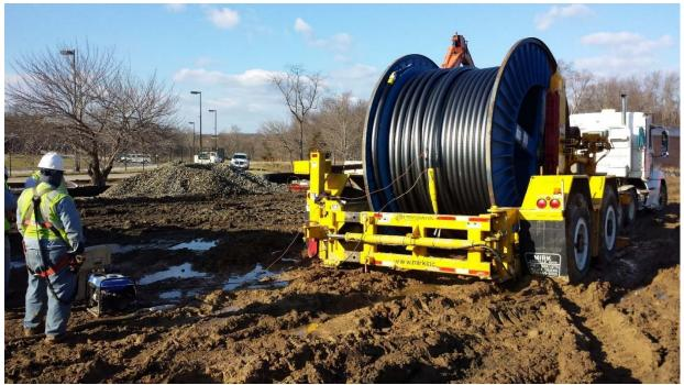
Figure 11 - Cable Reel Trailer
