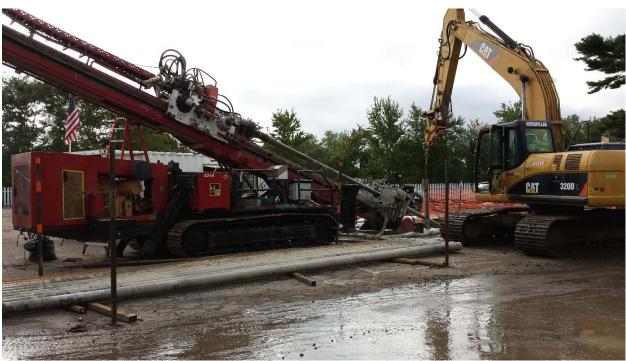
Figure 7 - HDD Drill Rig
