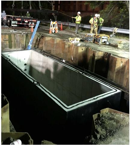
Figure 4- 115kV Splicing Vault
