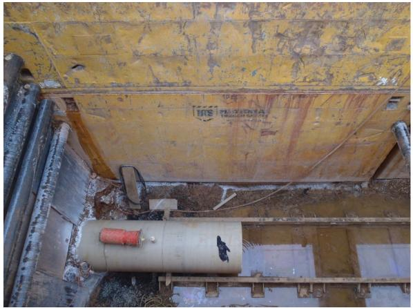
Figure 8 - Pipe Jacking Shaft
