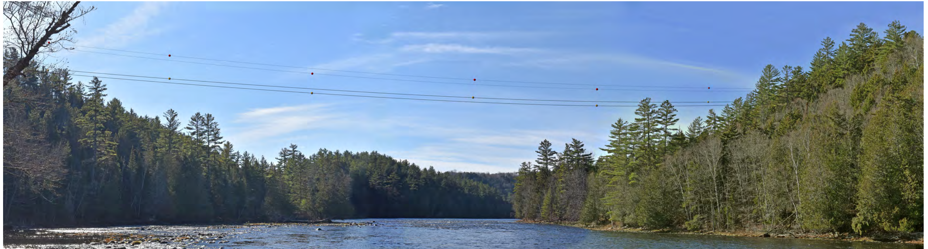
Proposed Conditions: Panoramic view looking from south to southwest from a point 750' +/- north of the proposed HVDC transmission line crossing of the Kennebec River near a rafting company picnic area. The closest structure, screened by vegetation in this view, is 850' +/- to the south. Conductors, approximately 200' above the river, will be visible to recreational boaters for approximately 1,600' approaching the crossing. Marker balls will be visible on the shield wires and conductors.
