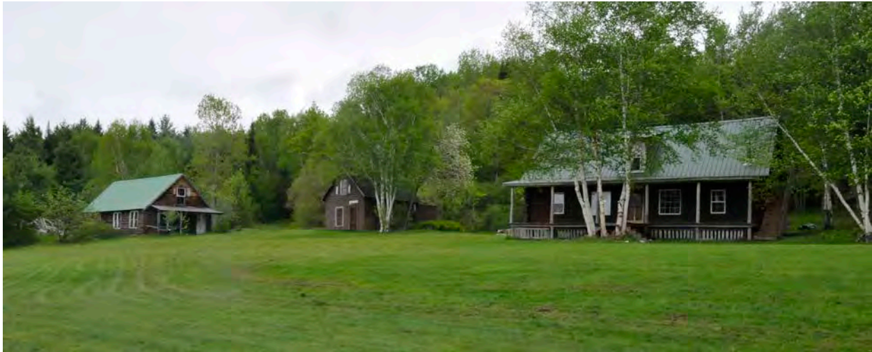
Several of the remaining structures at the Yexas Camps on Square Lake
