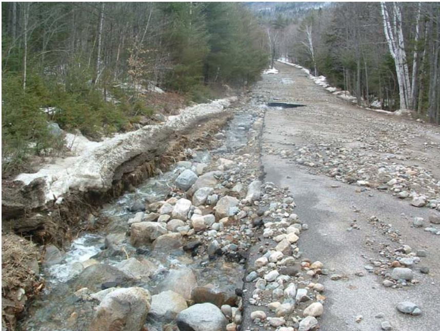
**Figure 43. Route 120 Washout in Andover Caused by Blocked Culvert, Maine April 5, 2005**
