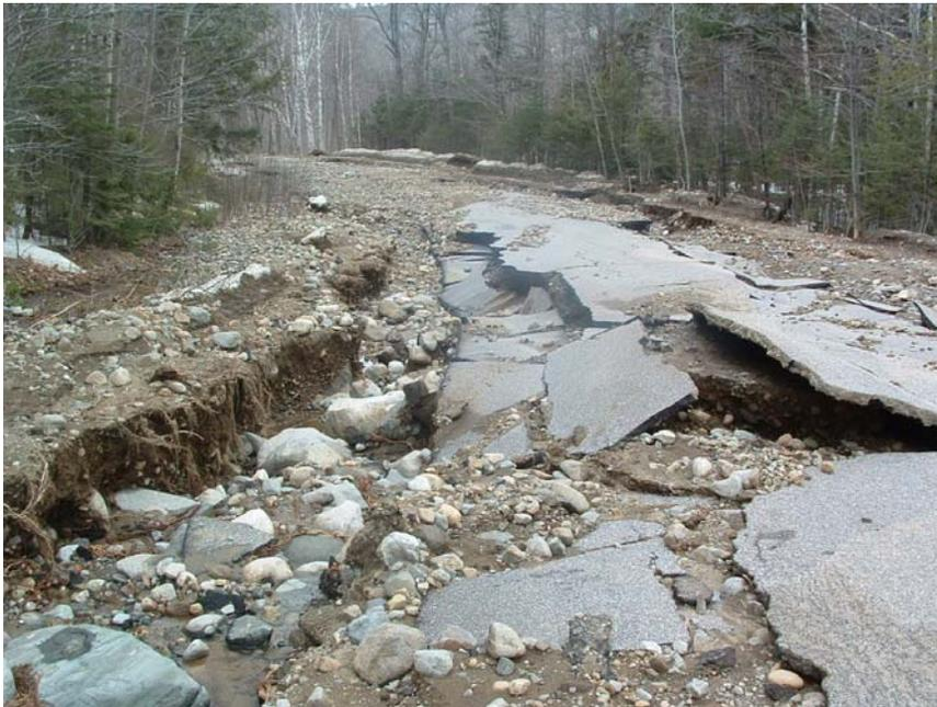
**Figure 41. Route 120 Washout in Andover Caused by Blocked Culvert, Maine April 5, 2005**
