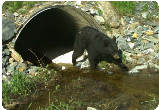
Above is an example of a wildlife habitat connector installed by the Maine Department of Transportation (MaineDOT) as part of the Caribou Bypass (Route 161) Project. Photo by MaineDOT.
