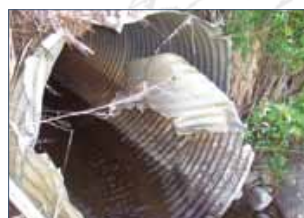
damaged culvert
