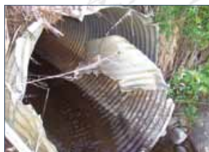
damaged culvert
