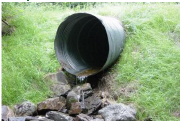
Perched and undersized culverts fragment stream habitat and restrict movement of fish and other wildlife
