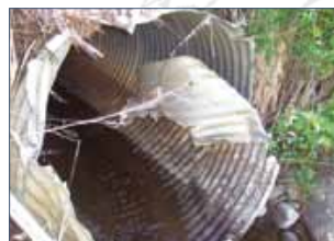
damaged culvert
