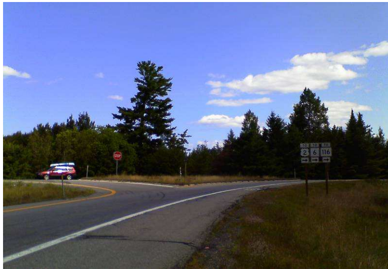
Northbound Off-ramp, Exit 227 – Lincoln, Maine
