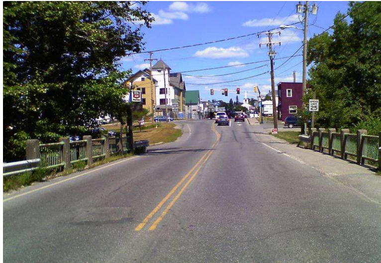
Narrow Bridge on Enfield Road (High Street), No Posted Restriction
