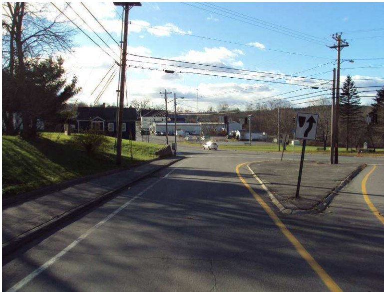
Intersection South Street & Route 1 – Calais, Maine
