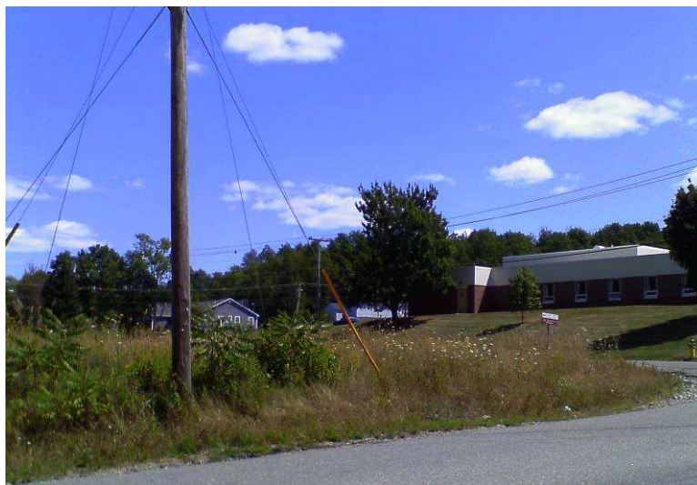
Guy on inside corner at Penobscot Valley Avenue & Route 115
