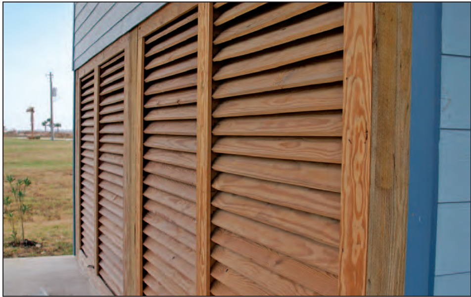
Figure 2-21. Louvers installed beneath an elevated house are a good alternative to breakaway walls
