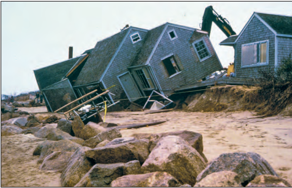
Figure 3-36. Undermined house at Chatham, MA, in 1988; nine houses were lost as a result of the formation of the new tidal inlet shown in Figure 3-35
