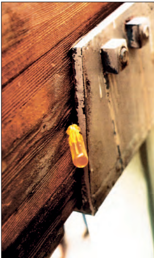
Figure 14-2. Wood decay behind a metal beam connector
