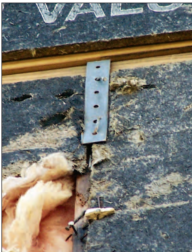
Figure 13-15. Connector failure caused by insufficient nailing
