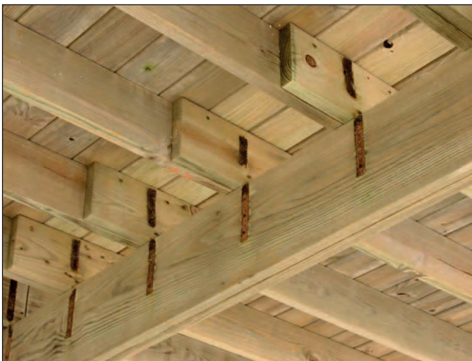
Figure 14-3. Severely corroded deck connectors
