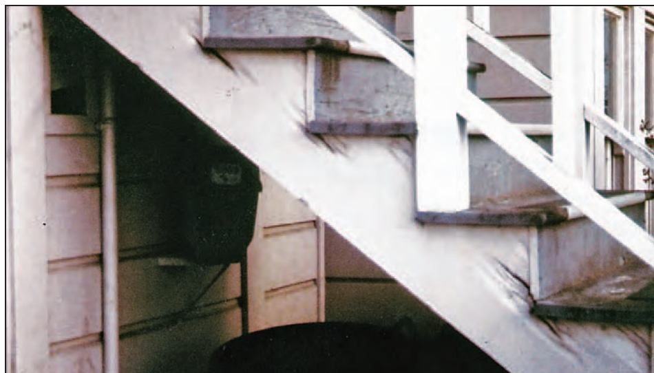
Figure 13-13. Deterioration in a notched stair stringer
