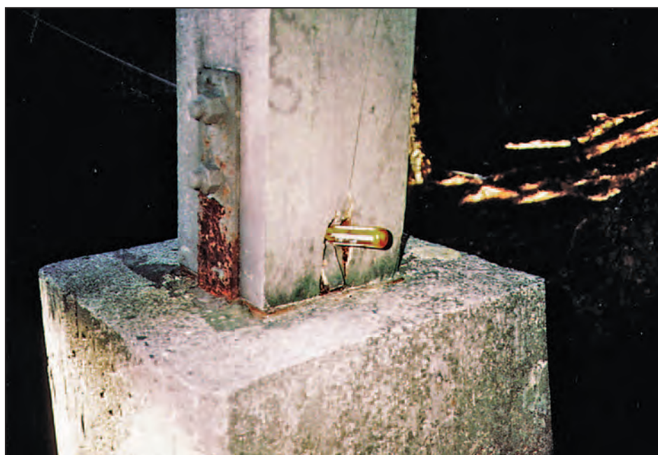
Figure 13-9. Wood decay at the base of a post supported by concrete
