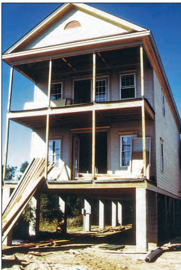
Figure 13-6. Open masonry foundation
