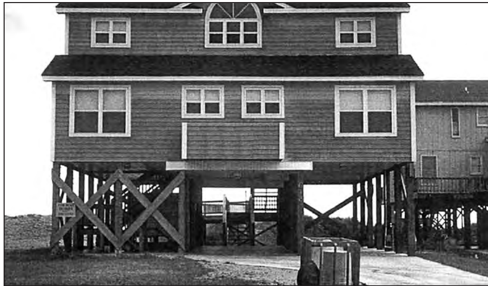
Figure 10-10. Diagonal bracing using dimensional lumber
