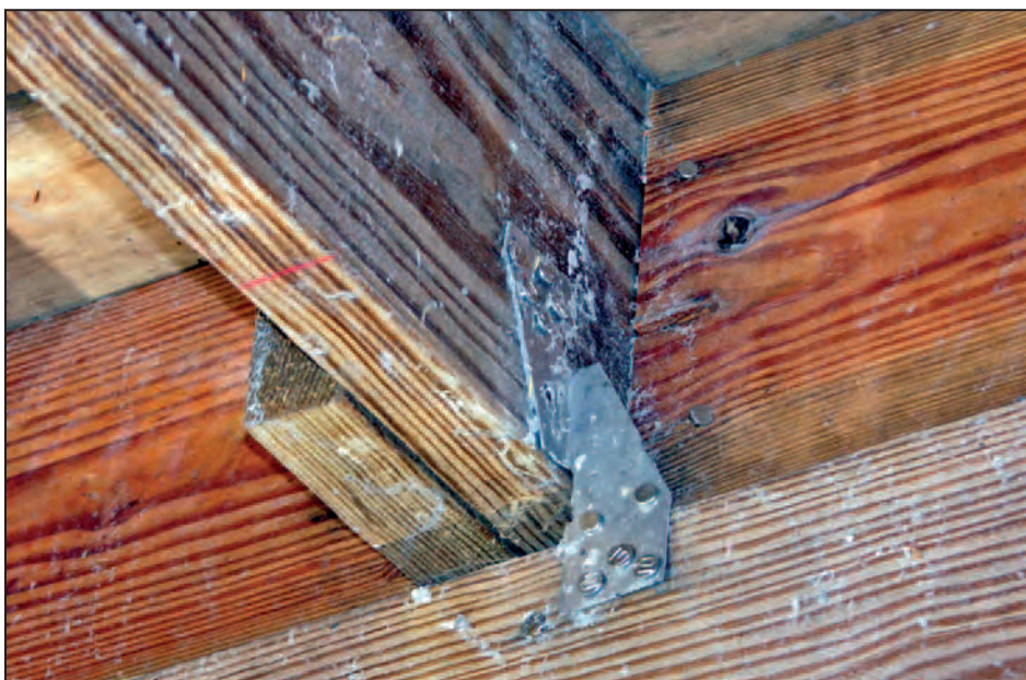
Figure 9-17. Metal joist-to-beam connector
