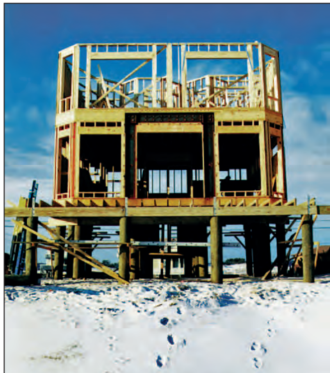
Figure 9-25. Steel moment frame with large opening
