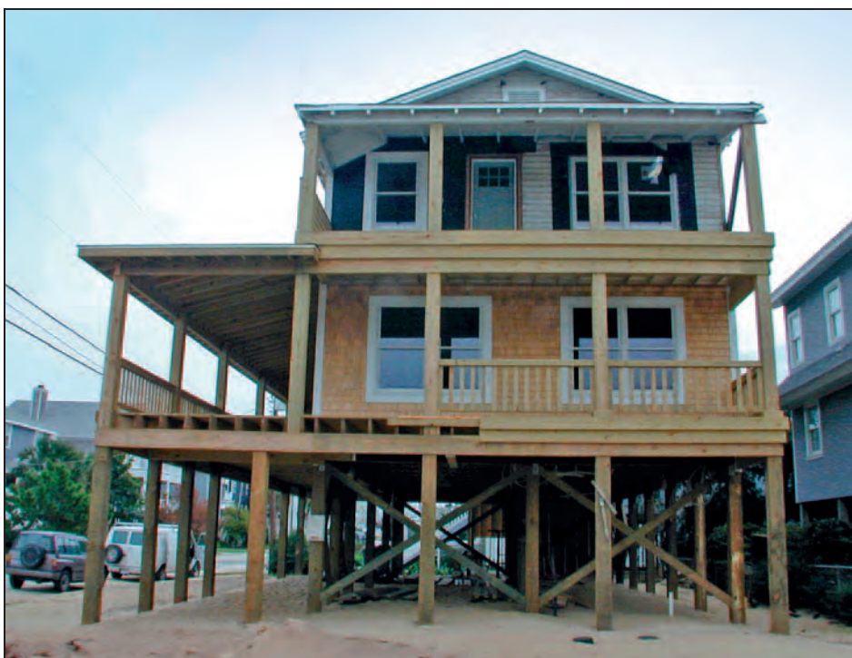
Figure 15-9. Home elevated on piles
