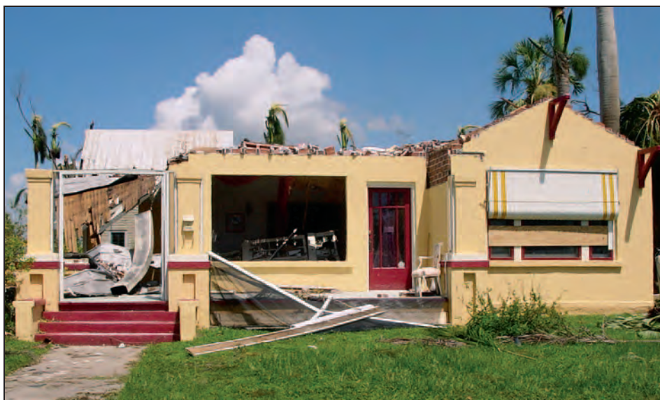
Figure 9-3. Roof framing damage and loss due to load path failure at top of wall/roof structure connection, Hurricane Charley (Punta Gorda, FL, 2004)
