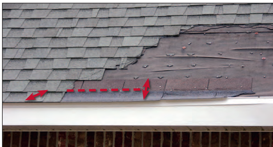
Figure 11-32. Incorrect installation of the starter course (incorrectly rotated starter, right arrow, resulted in self-seal adhesive not near the eave, dashed line). Estimated wind speed: 130 mph. Hurricane Katrina (Mississippi, 2005)
