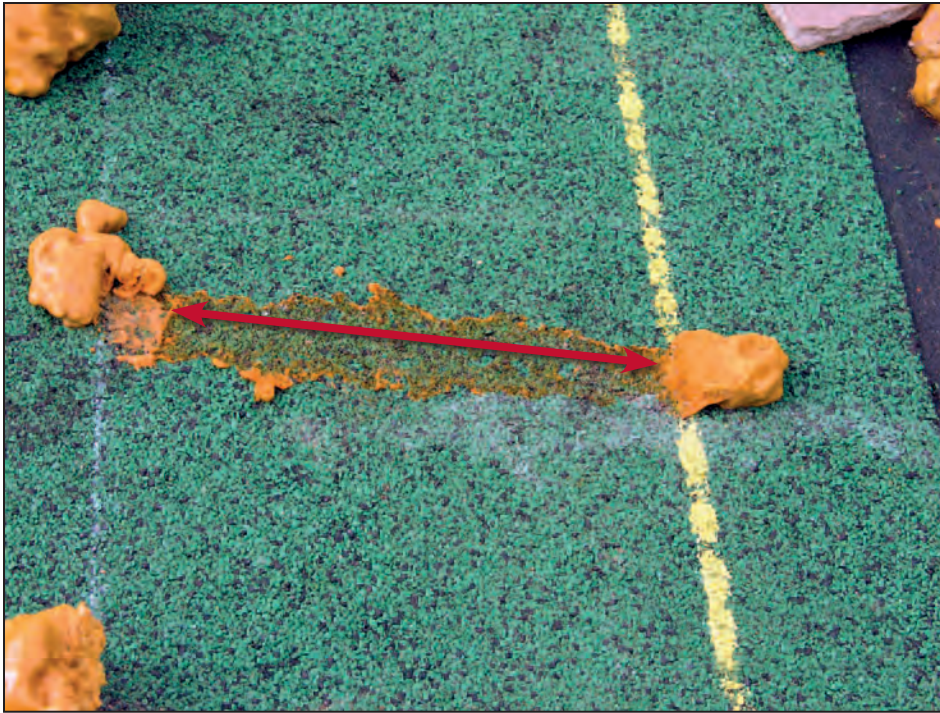
Figure 11-44. Adhesive that debonded from the cap sheet
