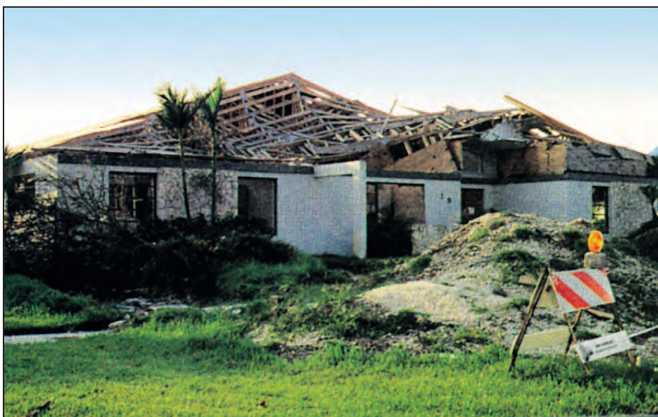
Figure 9-21. Gable-end failure, Hurricane Andrew (Dade County, FL, 1992)
